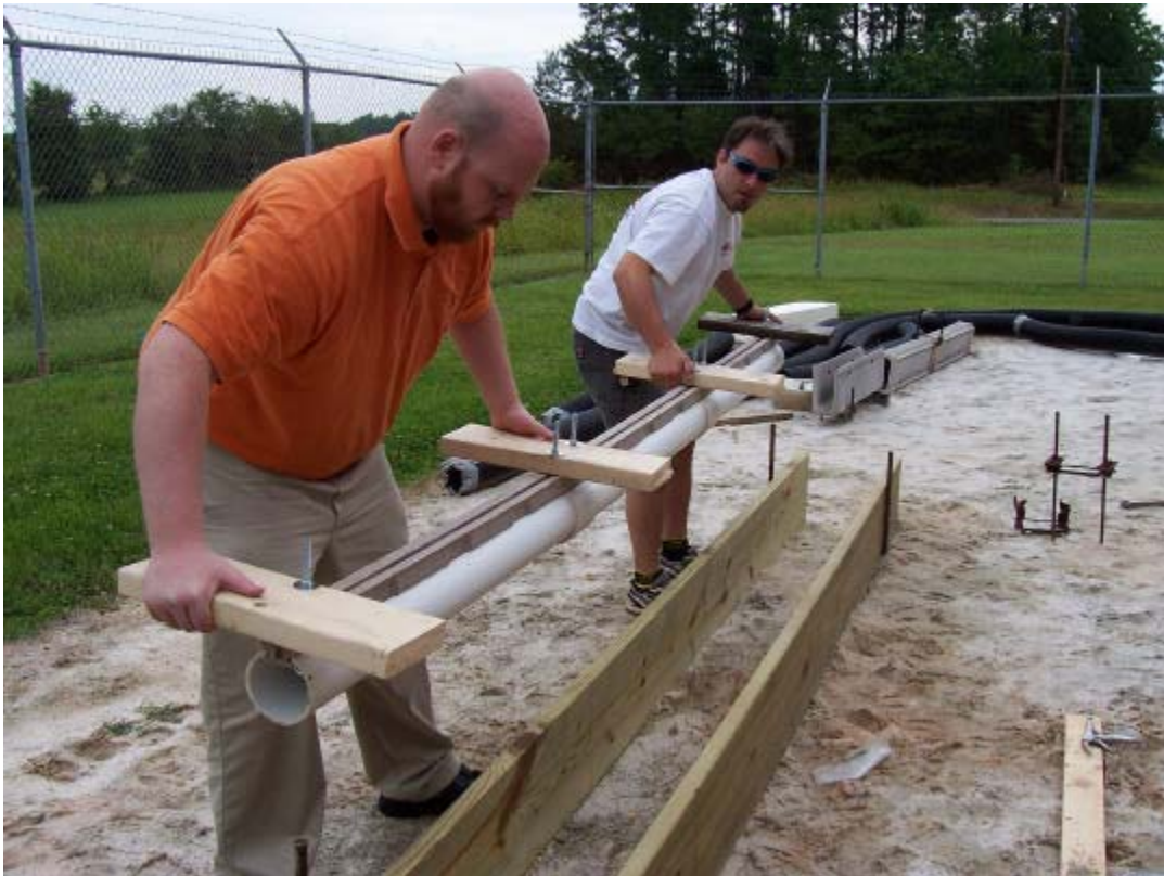
Sections may also be Pre-Assembled In Longer Lengths: EXAMPLE SHOWN: 3 Meters (9.84') Pre Assembled (51 lbs.)
