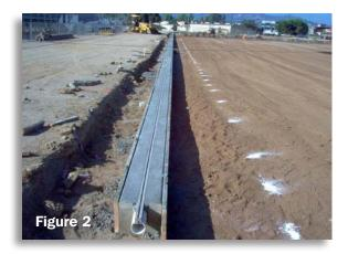
XT is manufactured of time tested and durable construction materials; polymer concrete and schedule 40 PVC. When properly installed and fully encased in concrete (see fig. 2), the product is virtually indestructible.
