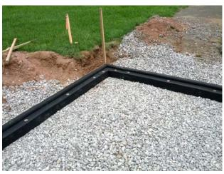
6. Using the pre drilled holes in the curb base drive the supplied 18 inch anchors into the ground. Follow the sight string line carefully, so the side of the curb is straight, not wavy. If one person places his foot (out of harm's way) on the curb, while the anchor is being installed, this will prevent the curb from moving and displacing the base.
