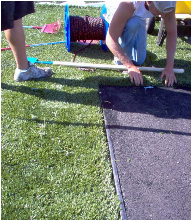
Rope Wedge Installation
