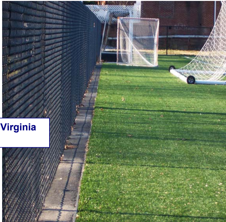
Turf Anchor Bordering a Stand Alone Infill Turf Field- Asphalt to Infill Turf
