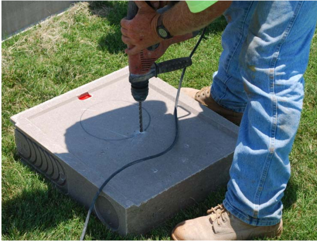
Typical 900 series catch basin installation
