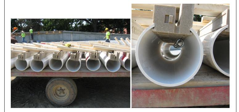
4. Place and center the assembled sections on the concrete forms. The high side of the XT-8 Collector should be oriented toward the track side. Make sure the XT-8 Collectors are set straight. The open polymer slot should remain aligned. The Collectors are joined end to end using the tongue-in-groove connection and the split PVC Joint Couplings. Nail suspension lumber to the edge forms. Once the drain is set and secured; double check the location and alignment before placing the concrete.
