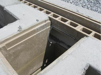
8. **Keep the drain slot openings protected** and clean throughout the construction process. Duct tape will help keep debris and concrete out of XT-8 Collector during installation.
