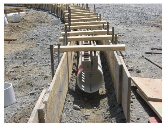
5. Before permanently setting catch basins, it is important to cut or drill out the appropriate 8" hole for the outlet pipe in the catch basin sidewall as indicated on the project design drawings. This can be done using a diamond tipped hole saw, or 3/8" masonry drill bit. When using masonry drill bit, drill holes around the circumference at 3/4" centers and tap out the remaining fins of polymer concrete with a cold chisel.
