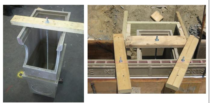
7. The catch basin assembly can now be set on the form placed for them so that the catch basin fits tightly against and conforms to the XT-8 Collector. Reach inside the catch basin top and trace the perimeter of the visible PVC pipe. Lift the basin assembly out and **cut out the traced hole** with the appropriate saw. Place the basin assembly back on the forms and secure. Make sure the catch basin is positioned snugly against the PVC pipe and polymer concrete top of the XT-8 Collector.
